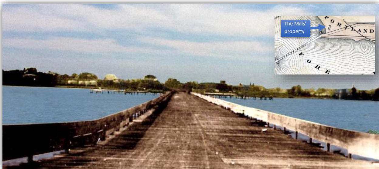
A colorized photograph of the 1,300-foot Vaughan’s bridge and its planking, looking from Portland across the Fore River
